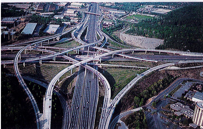
FIGURE 7 An all-directional interchange is used in complicated intersections with high-volume traffic. From this interchange, traffic is channeled in many different directions.
