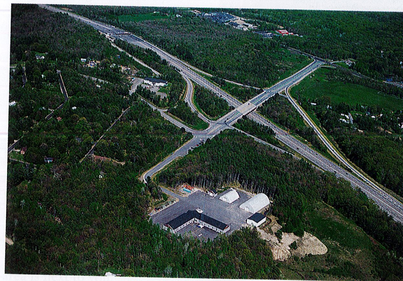
FIGURE 5 A diamond interchange is used when a road that crosses a busy highway has little traffic.
