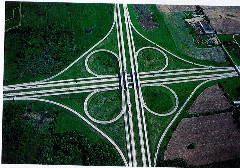
FIGURE 4 A cloverleaf interchange has a series of entrance and exit ramps that resemble the outline of a four-leaf clover. This type of interchange enables drivers to proceed in either direction on either highway.
