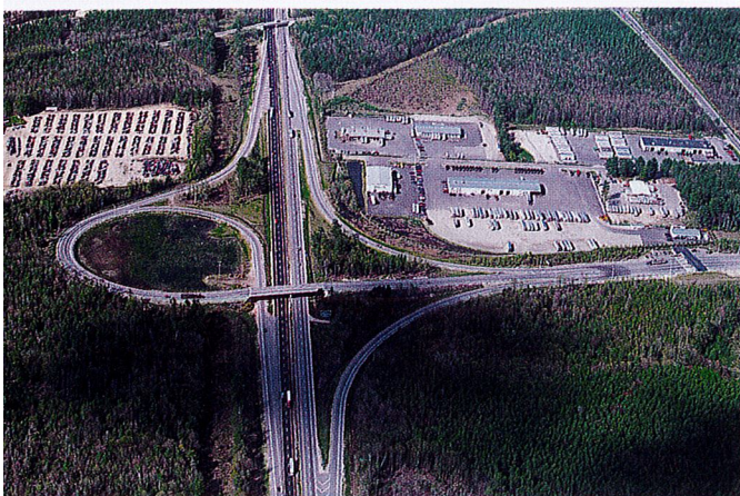
FIGURE 6 A trumpet interchange is used where one highway forms a T-intersection with a freeway.
