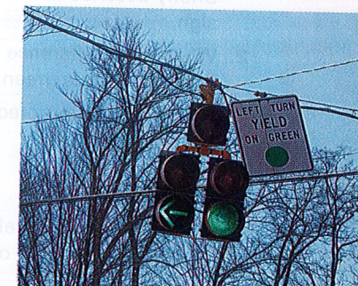
FIGURE 10 This traffic signal is called a "doghouse." The green arrow permits you to make a protected left turn.
