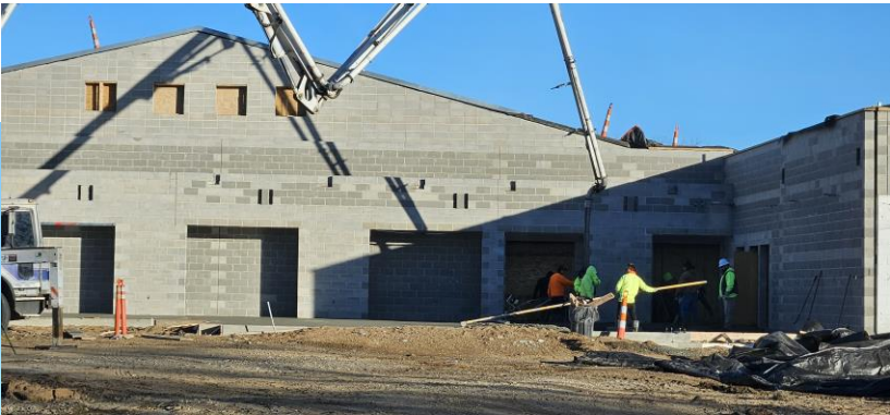
Concrete has been poured and beams are being installed....
