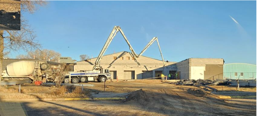
Concrete has been poured and beams are being installed....
